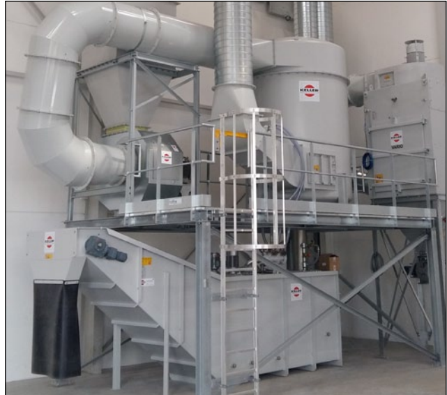
Wet scrubber VDN-TA with sludge remover
