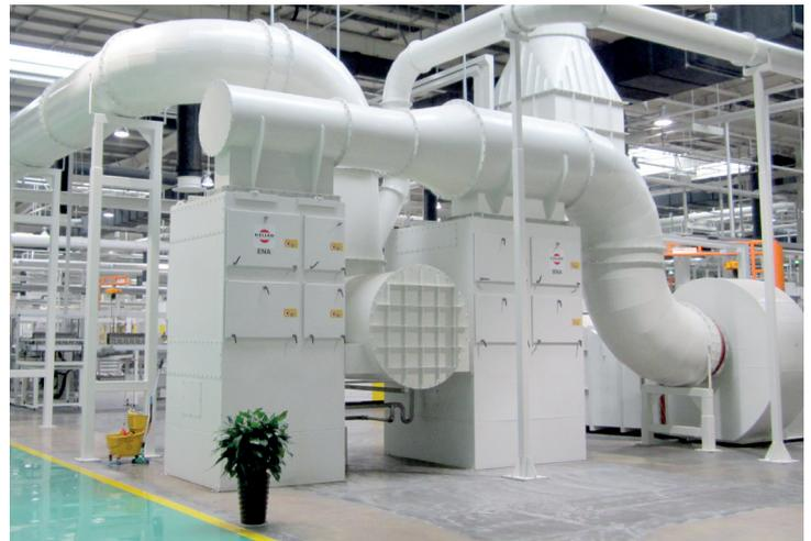
Dust extraction of a truck-engine production with a volume flow of 140 000 m<sup>3</sup>/h
